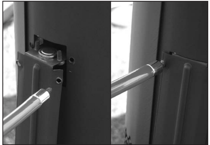
Figure 43: Spill switch installation.
